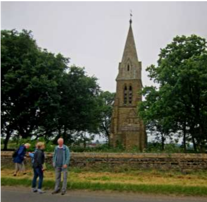
Walkers stop to examine this ruined church spire at Little Brington.
